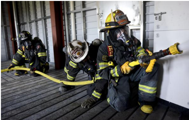
Figure 4—Live Burn Building, Typical
