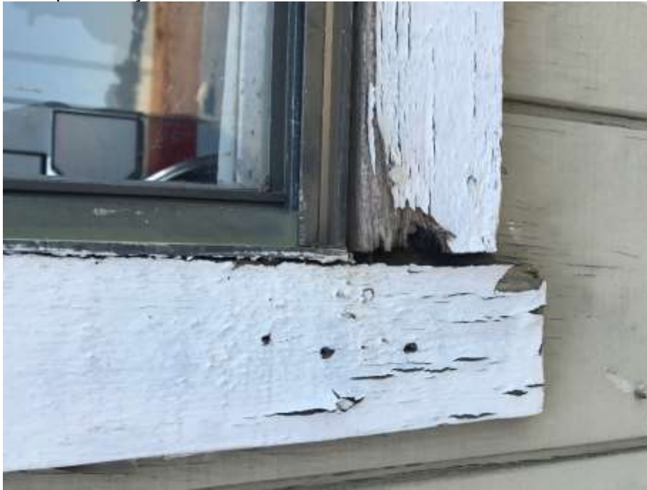
Example of Dry Rot On Exterior
