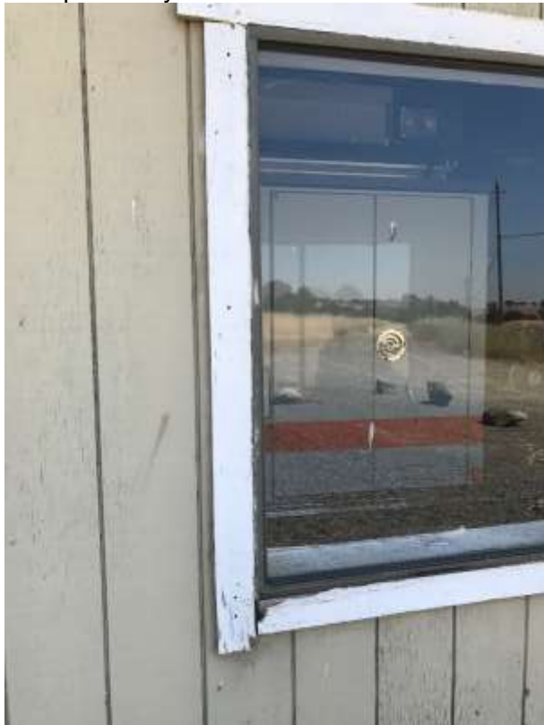
Example of Dry Rot On Exterior
