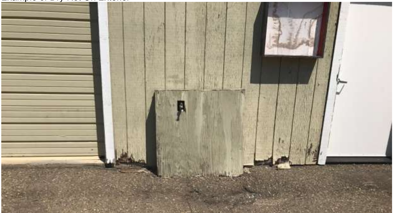
Example of Dry Rot On Exterior
