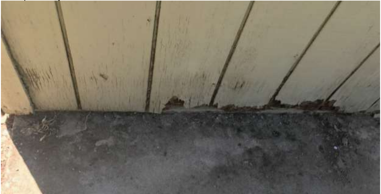
Example of Dry Rot On Exterior
