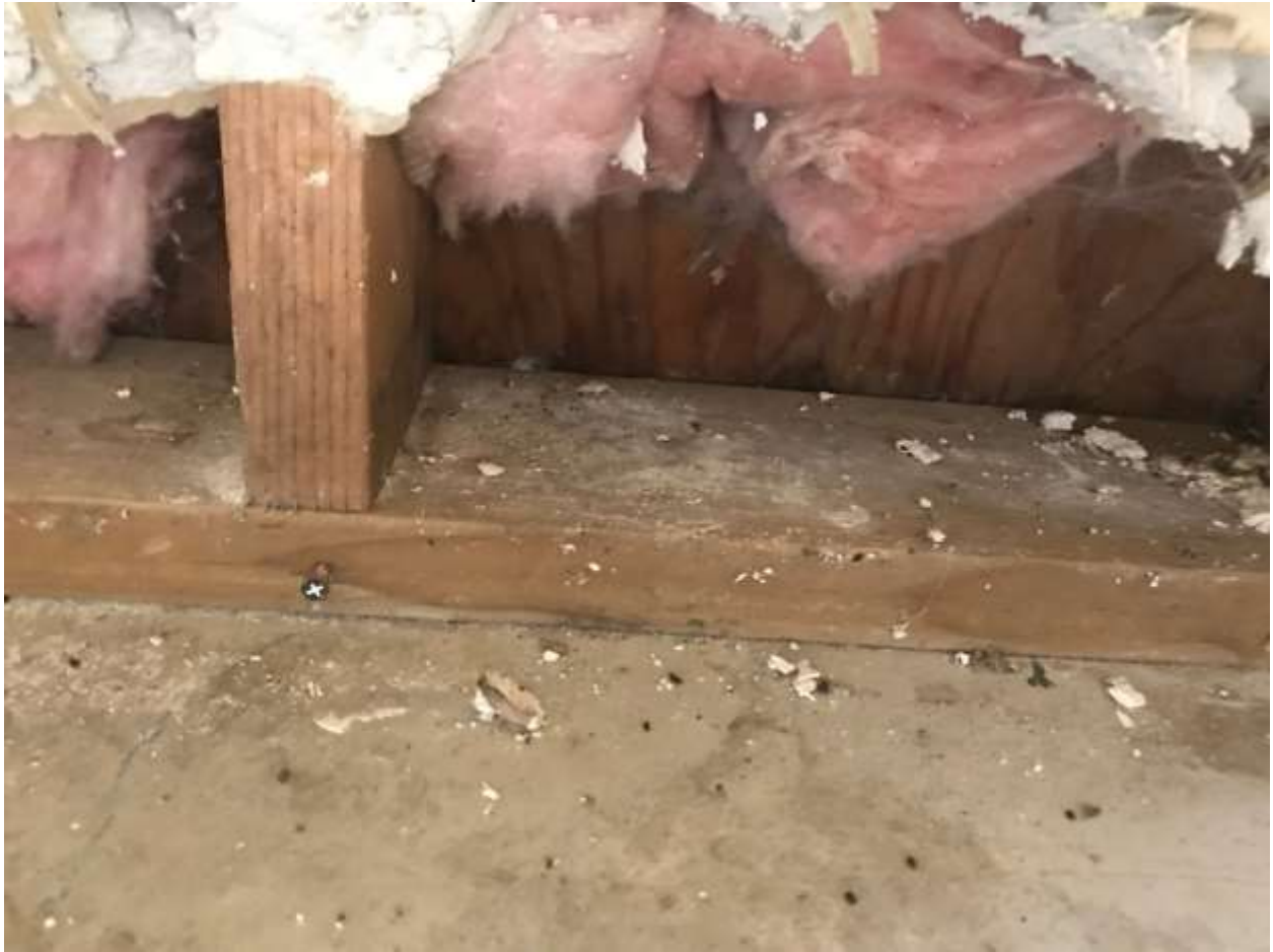
Interior Construction – Lacks Waterproof Membrane
