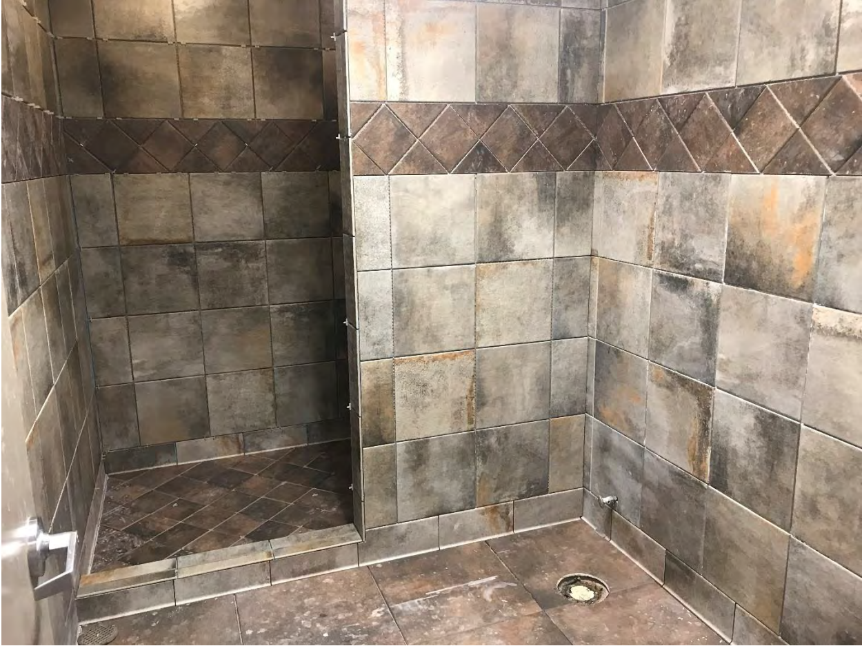
Station 86 Bathroom Remodel Underway. 3/29/18 Photo
