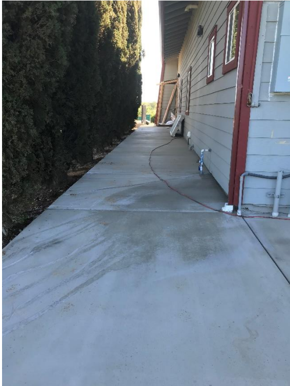
New sidewalk – Southside of Station
