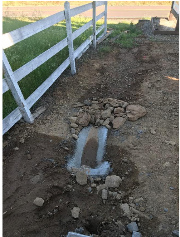
New Drainage Outlet
