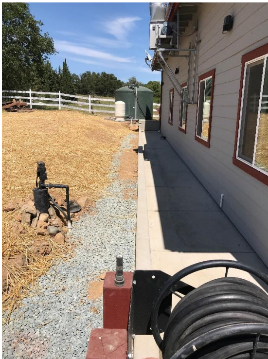
New Drain – Northside of Station
