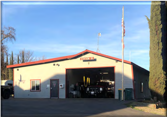
Station 91 (Latrobe), 7660 South Shingle Road. Shingle Springs, CA 95682
