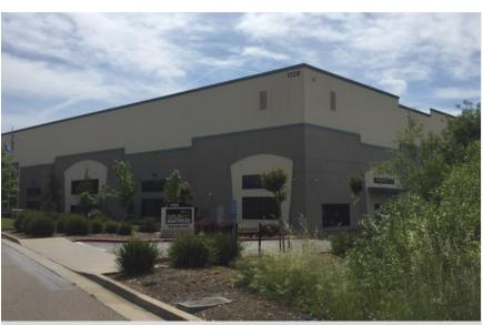
Tilt-up construction, as shown in this example, often have large expanses of open space where fires can spread, flashover is more intense, roof ventilation is required to remove smoke, and firefighters can easily lose their sense of direction in the smoke.
